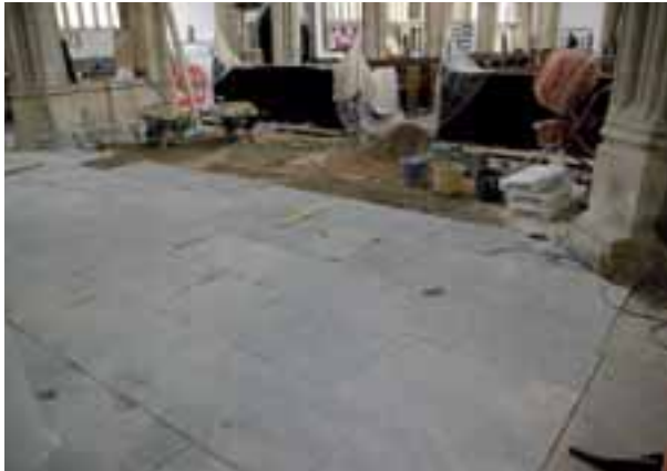
Work in progress on the new blue lias flooring
