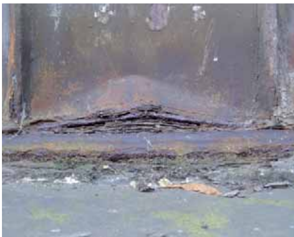
Corroded shim
