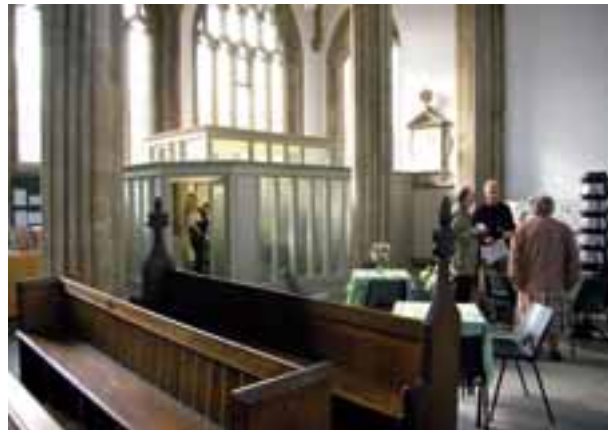
The completed Parish office
