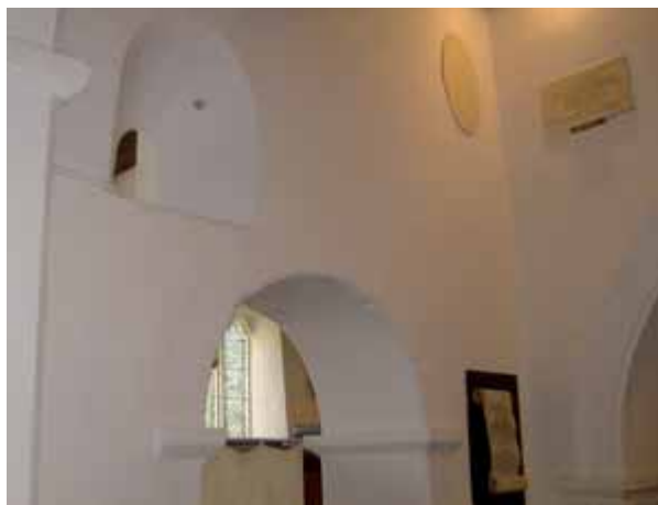
Inside St Mary's Saxon tower
