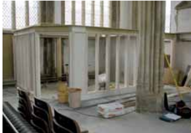
Parish Office under construction
