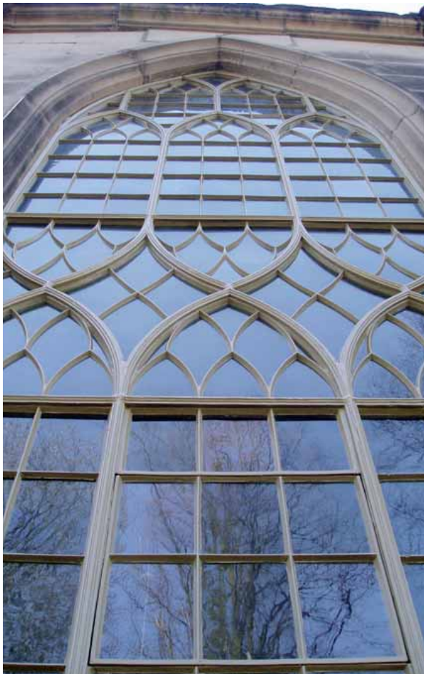
NW window after repair
