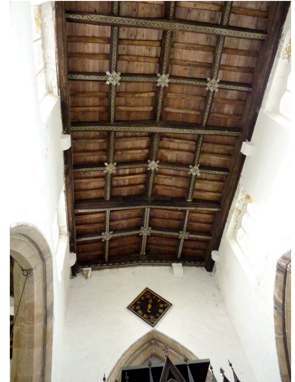
The completed roof from below.
