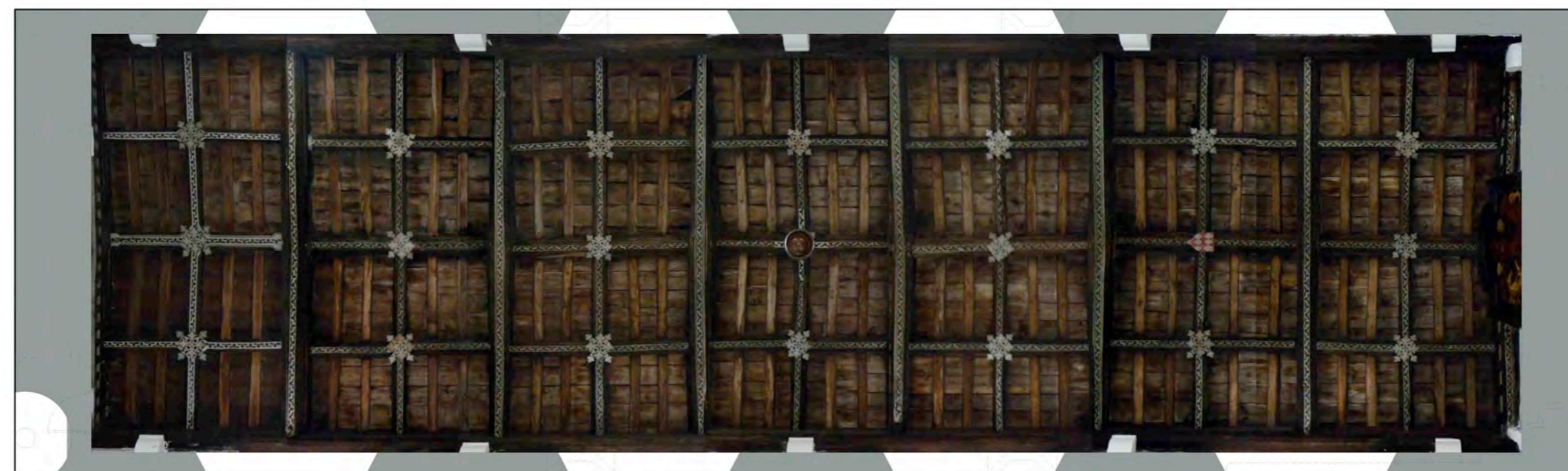
Survey photograph of roof structure prior to works
