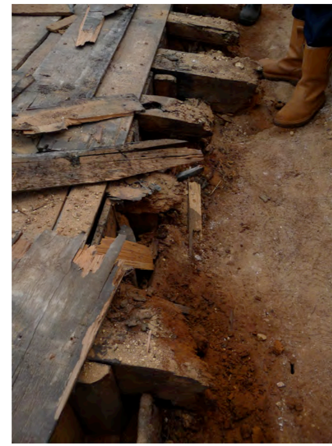
Typical condition of beam and rafter ends. The remains of the wall plate could be removed with a vacuum cleaner.
