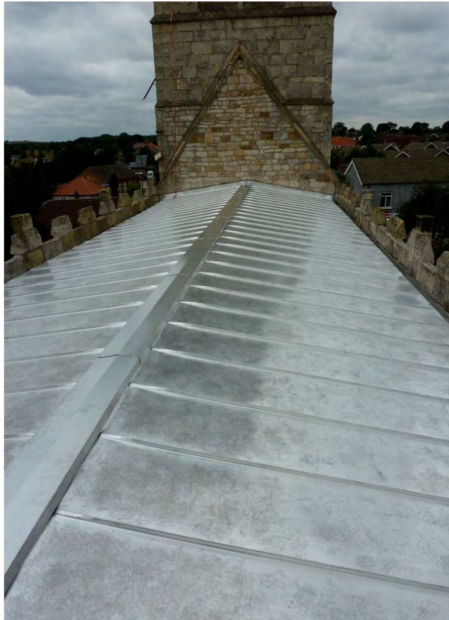
The complete roof.
