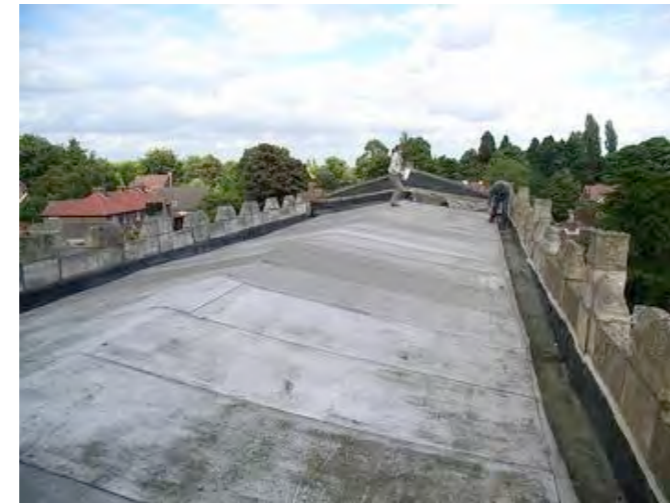
Existing asphalt roof coverings. The gutters were poured asphalt.
