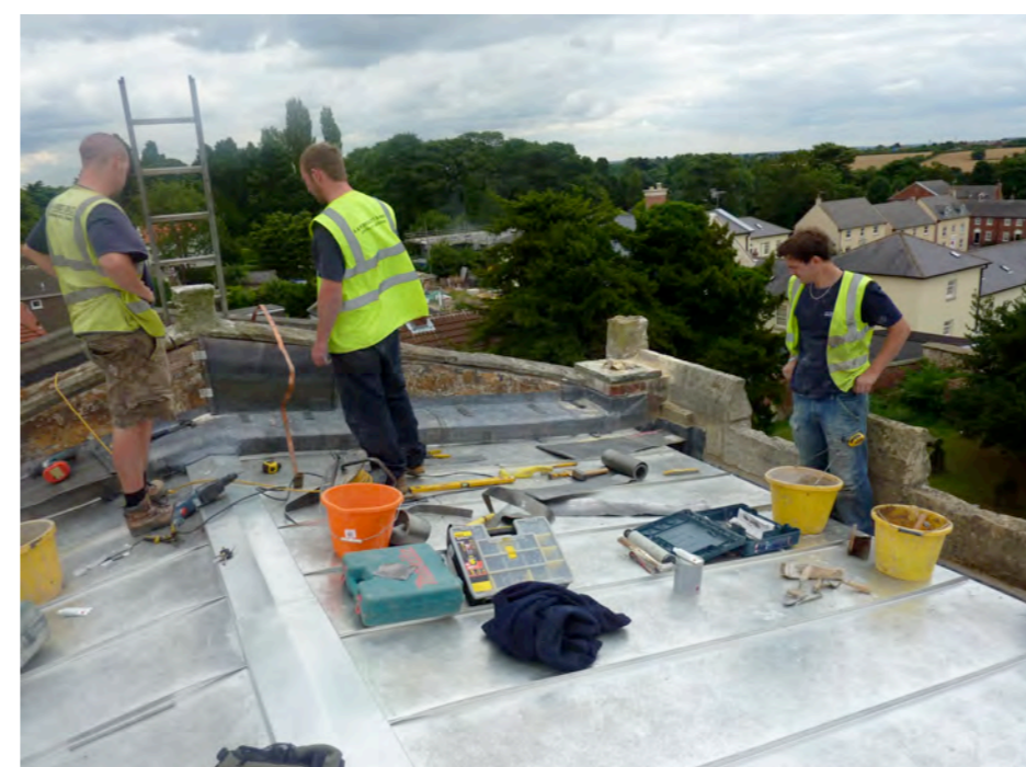
Photograph showing that the finished roof line is only 150mm above the original line.
