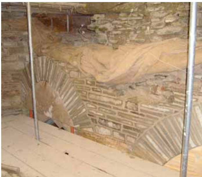
Rebuilding the arches
