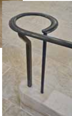
Iron handrail detail
