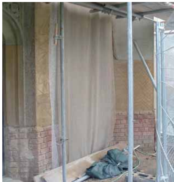
Re-rendering works in progress together with reduction in ground levels
