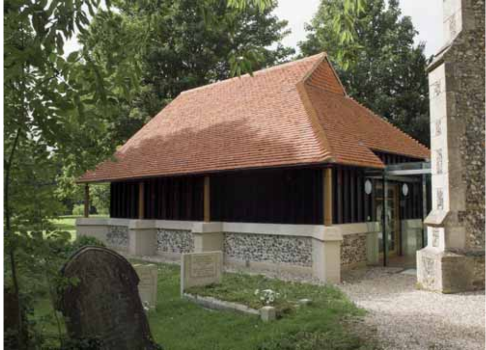
View from the south east
