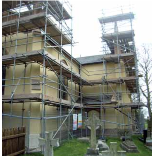
Repair works to renders and pinnacles
