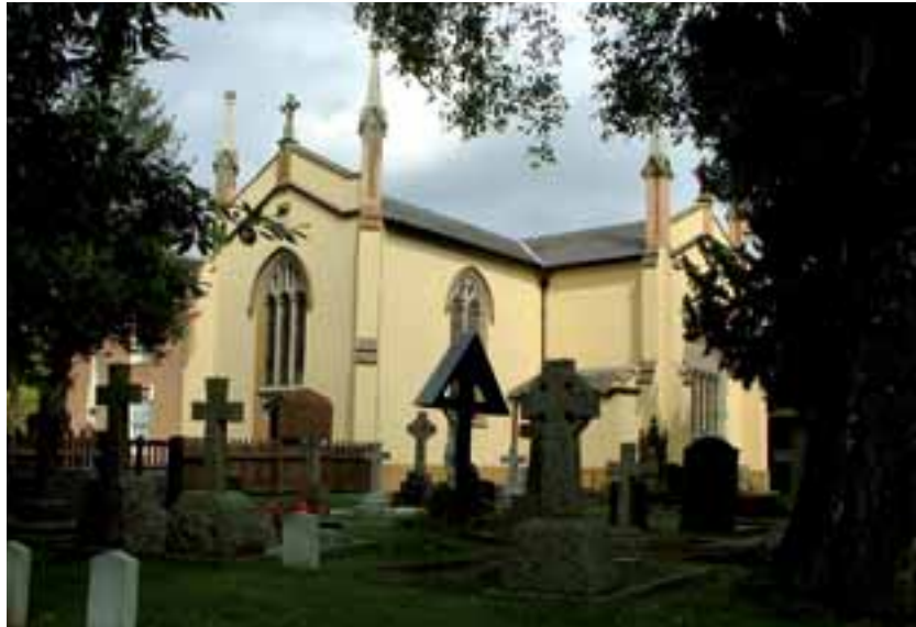
View of completed works from the south west corner of churchyard
