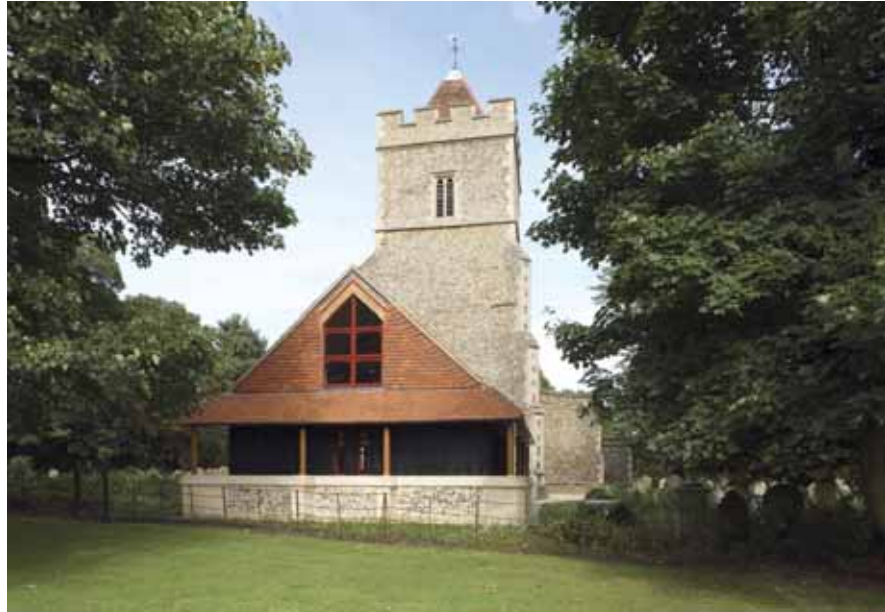
View from the west
