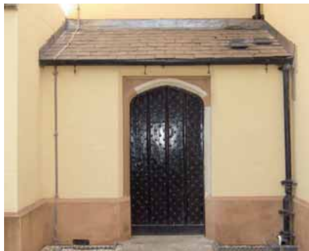
Completed repairs to renders and lean-to roofs
