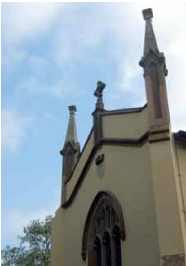
View of completed pinnacles at west end
